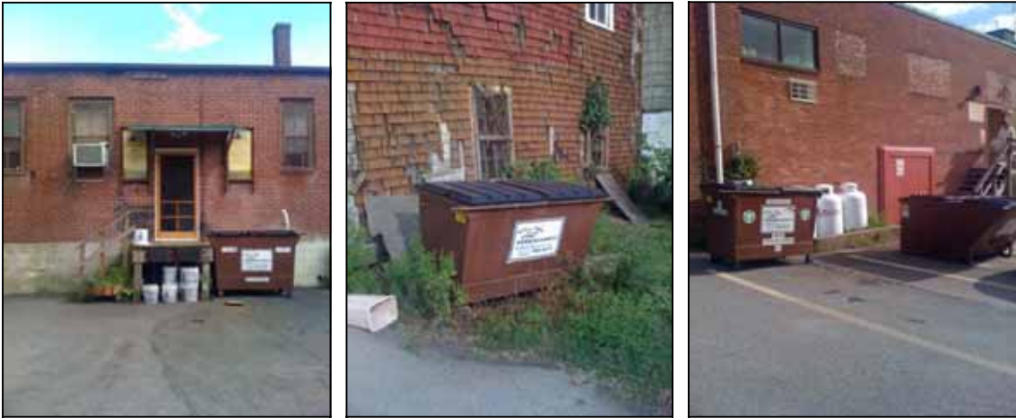
These unscreened dumpsters characterize the use of private land abutting the public lot.
