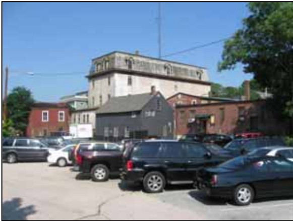
View of the Saugatucket Parking Lot from Saugatucket River Walkway.
