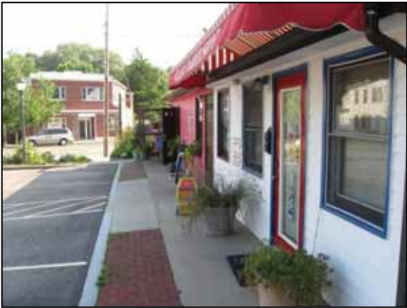
The building edge abutting the public lot exhibits many pedestrian elements.
