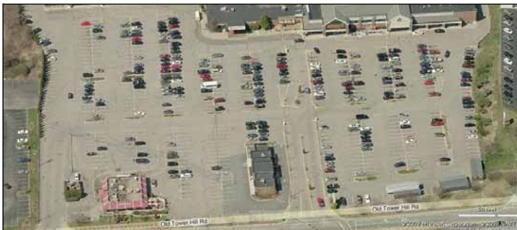
Development within Dale Carlia is dominated by vast amounts of asphalt, such as the Wakefield Mall shown here.
