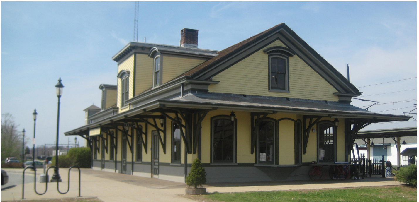
Historic Kingston Station
