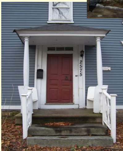
Colonial Revival: 1890-1940 return to Colonial forms, porches with Tuscan columns and benches, enlarged doorway trim
