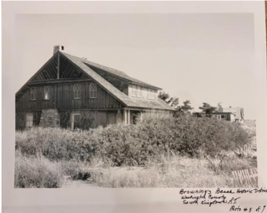
NR Nomination, 1997, view to northeast
