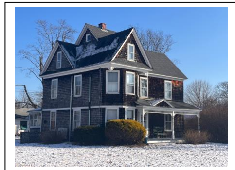
Photo ID SOKI WashingtonSt0011 SE
