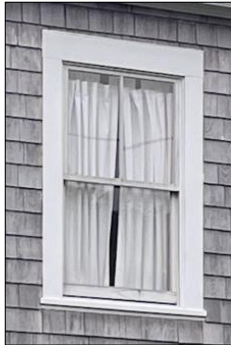
Figure 23. A 2/1 double hung wood window at 47 Atlantic Avenue.
