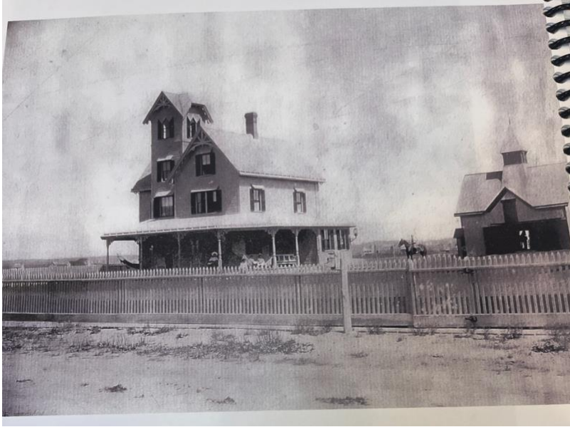
Undated photograph, showing south and east elevations, view to northwest.
