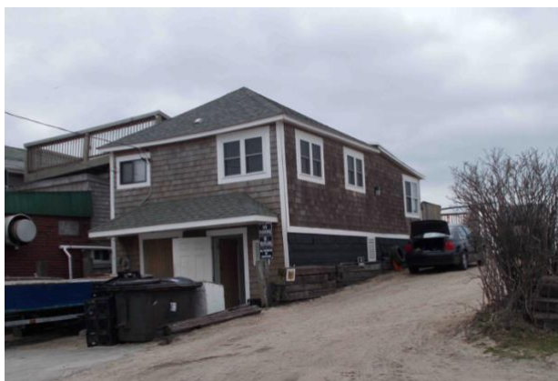
Photograph, 2024, of second building on parcel, showing the south and west elevation, view to the southeast.
