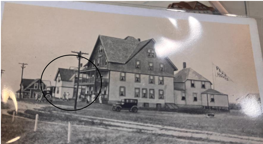
Undated photograph, view to northwest, collection South County History Center
