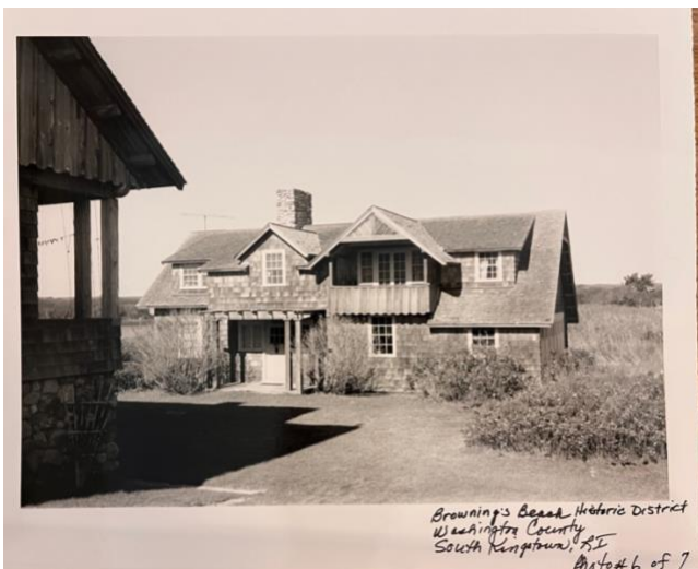
Photograph, NR nomination, 1997, view to northwest. After it was elevated on piers in 2009, there were several notable modifications, including adding a gabled portico, wrap-around deck, the change of fenestration in bays 1 and 3 from windows to double doors, and the addition of double doors on the west and east elevations.
