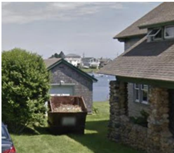
2012 photograph, view to southeast, Google Streetview, 2025
