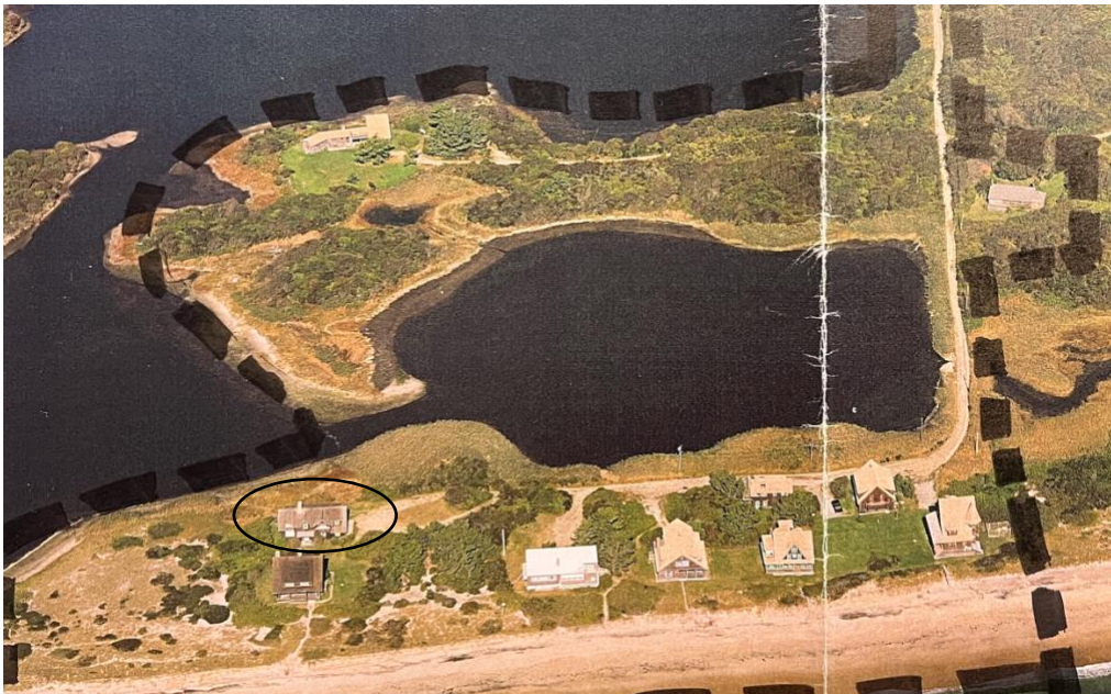
Aerial image, NR Nomination, 1997, showing Knight-Bontecou Carriage House/Garage (oval in lower left).
