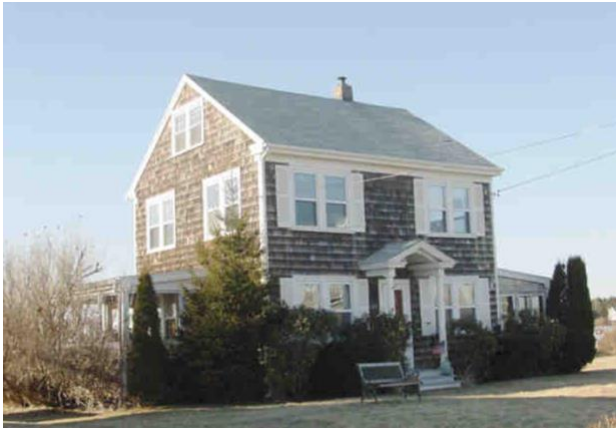
Undated photograph, view to northwest, showing more clearly the side wings, South Kingstown Tax Assessor
