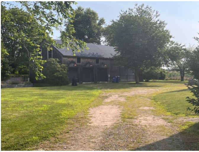
Photograph of barn, 2024, survey photo, view to northeast
