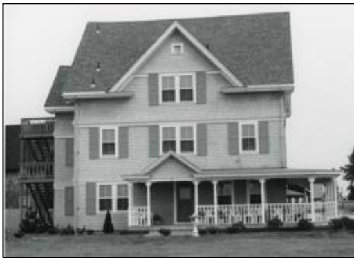
Figure 66. Dewey Cottage, 1989, NR Nomination, view to east. (left)
