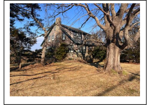
Photo ID SOKI PeninsulaRd0108 N
