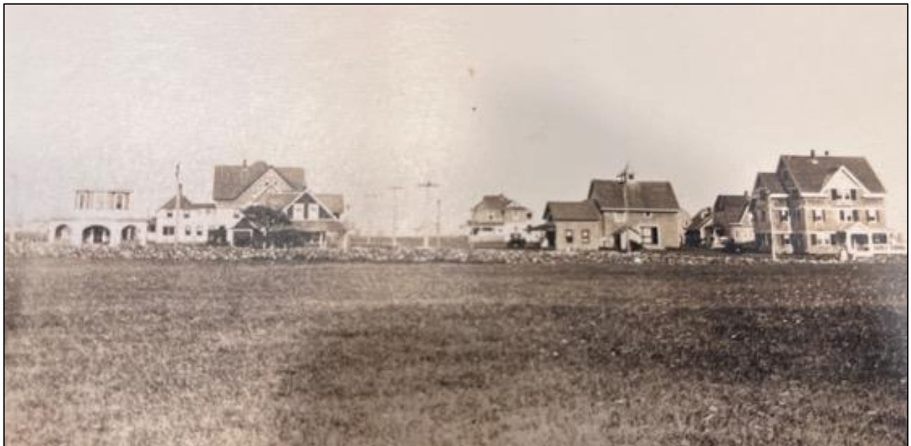
Figure 9. Matunuck Park, 1916 photograph, looking east from the Lower Weeden Farmhouse (now 65 Blackberry Hill Drive), showing Allview Cottage (Barney's Pagoda), Park Hotel, Clark House, Briggs Cottage, and Dewey barn and Cottage (left to right), collection South County History Center.
