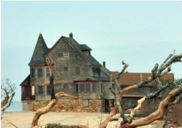
Photograph, June 13, 2013, credit Michael Derr for The Independent, showing house after Hurricane Sandy (2012) and prior to subsequent relocation and elevation on concrete piers, view to southwest
