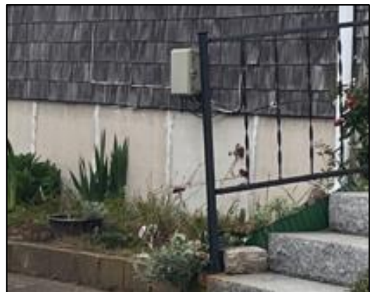
Figure 24. 40 Prospect Road, built 1923, Detail, showing a non-historic poured concrete foundation.
