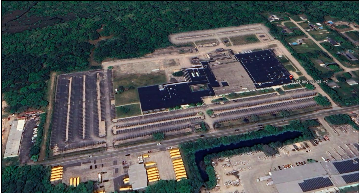
Figure 4 – On-site, existing conditions – underutilized, impervious parking area to note
