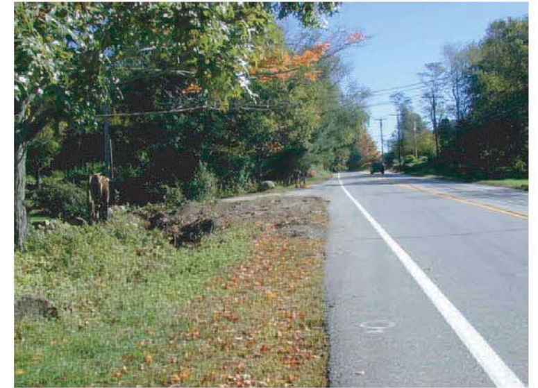
Roadway and Shoulder
