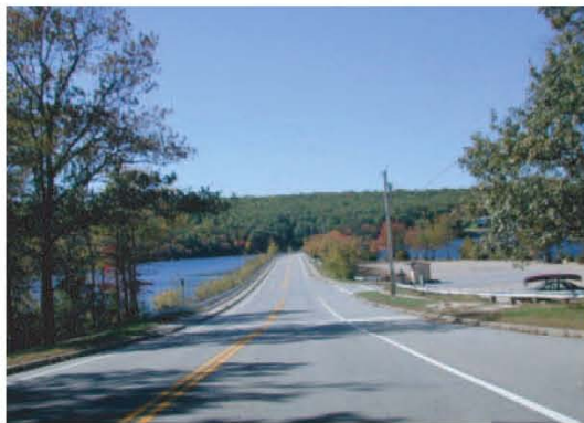
Route 165 approaching Connecticut at Beach Pond
