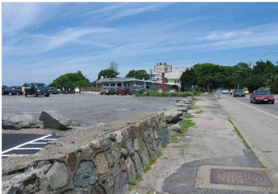
Road edge at the Northern Threshold
