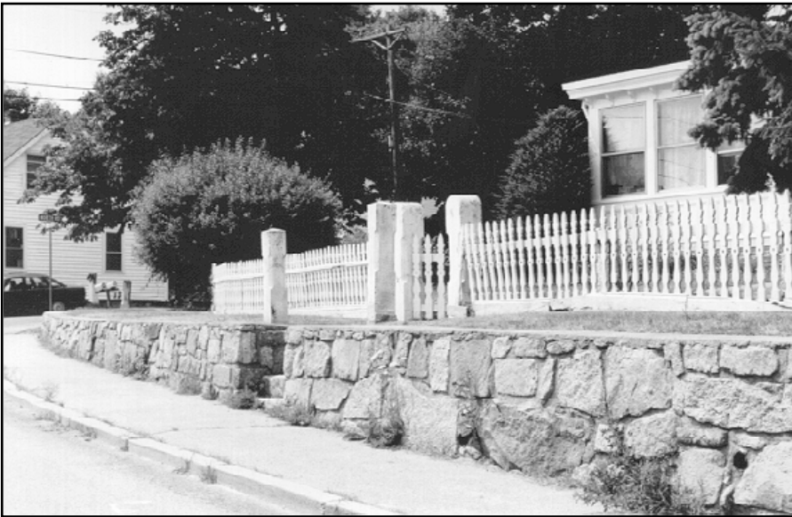
Fencing provides interest and continuity throughout the village.
