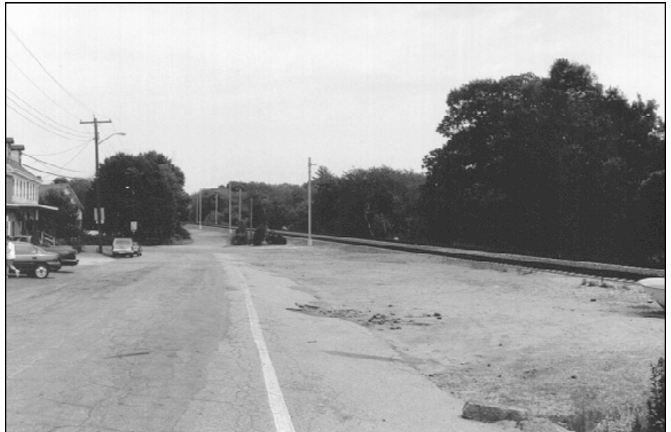
Power lines will rise above the railroad visually defining the narrowness of the roadway.
