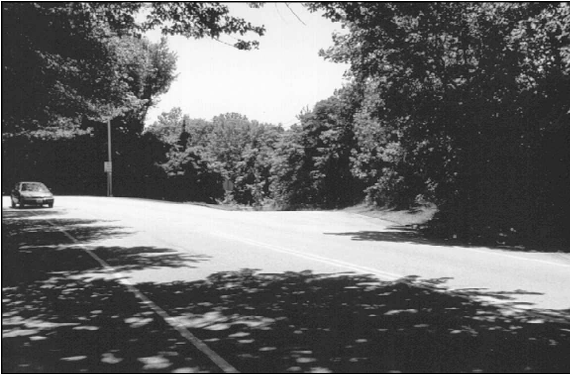
The intersection of the Kettle Point access road with Veteran Memorial Drive is dangerous.
