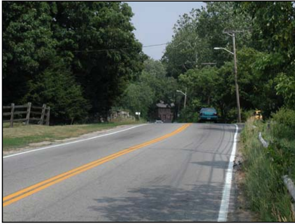
Great Road - looking east
