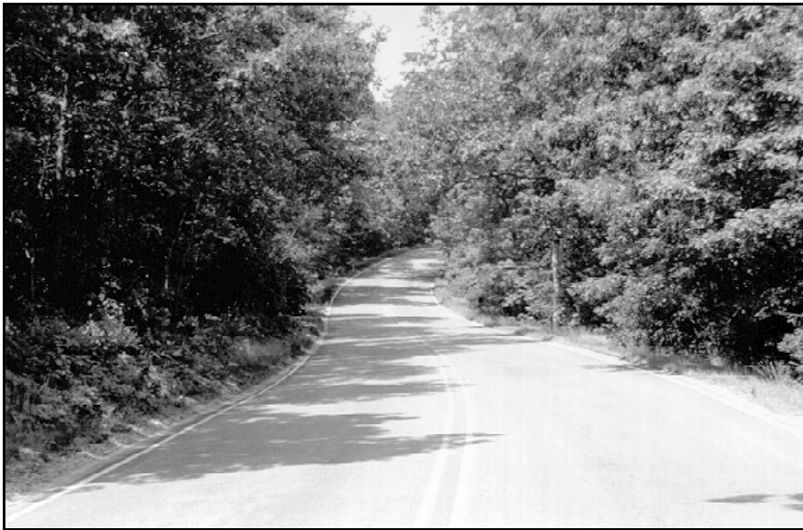
Roadway management should focus on protecting the width, alignment and rural character of the road.
