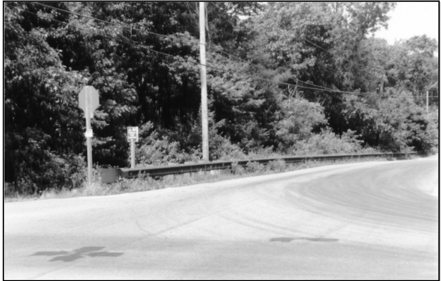
Today's galvanized guardrail at Tuckertown Four Corners.
