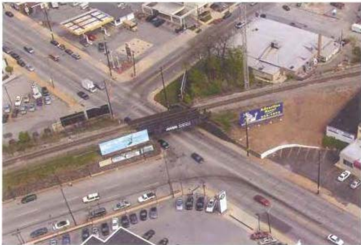
Plate 028 CSX railroad overpass at Pennsylvania Avenue
