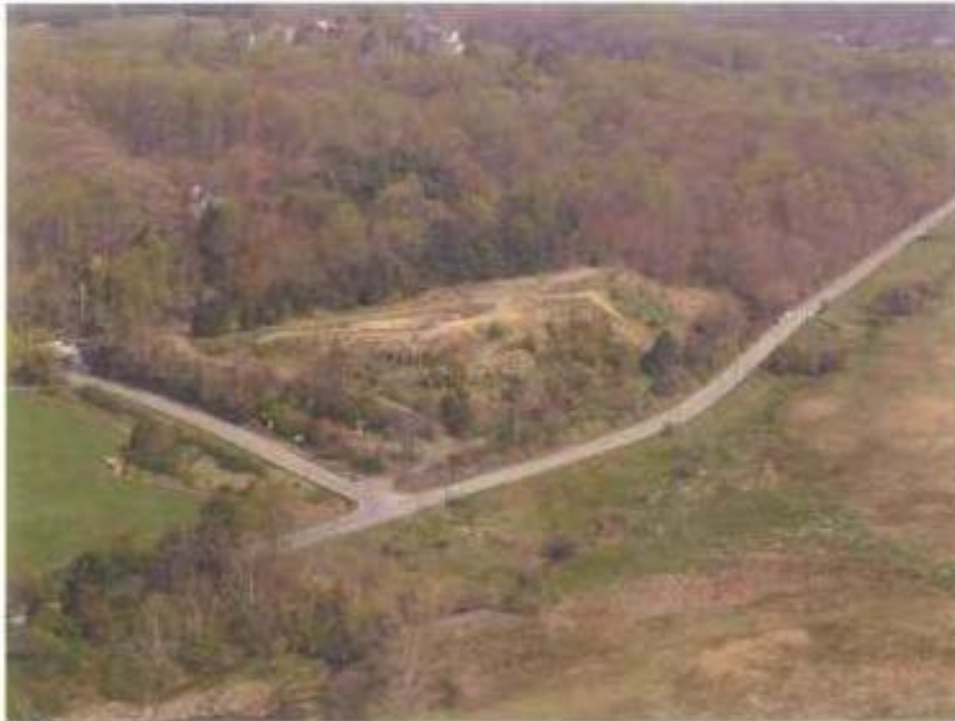
Plate 107 Rubble mound from the air
