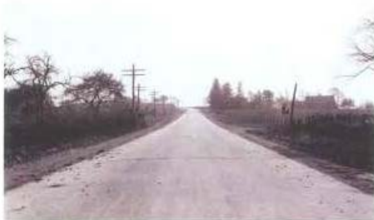
Plate 084 Kennett Pike south from the state line near the Line House, ca. 1910
