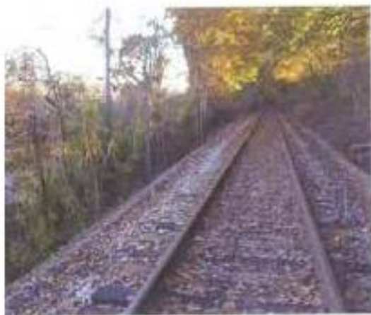
Plate 102 Wilmington and Northern railroad and its right-of-way
