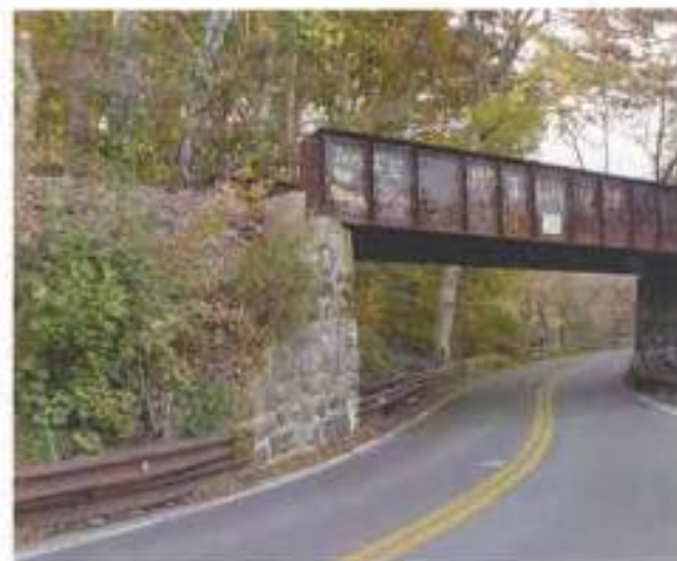
Plate 098 Wilmington and Northern railroad overpass.
