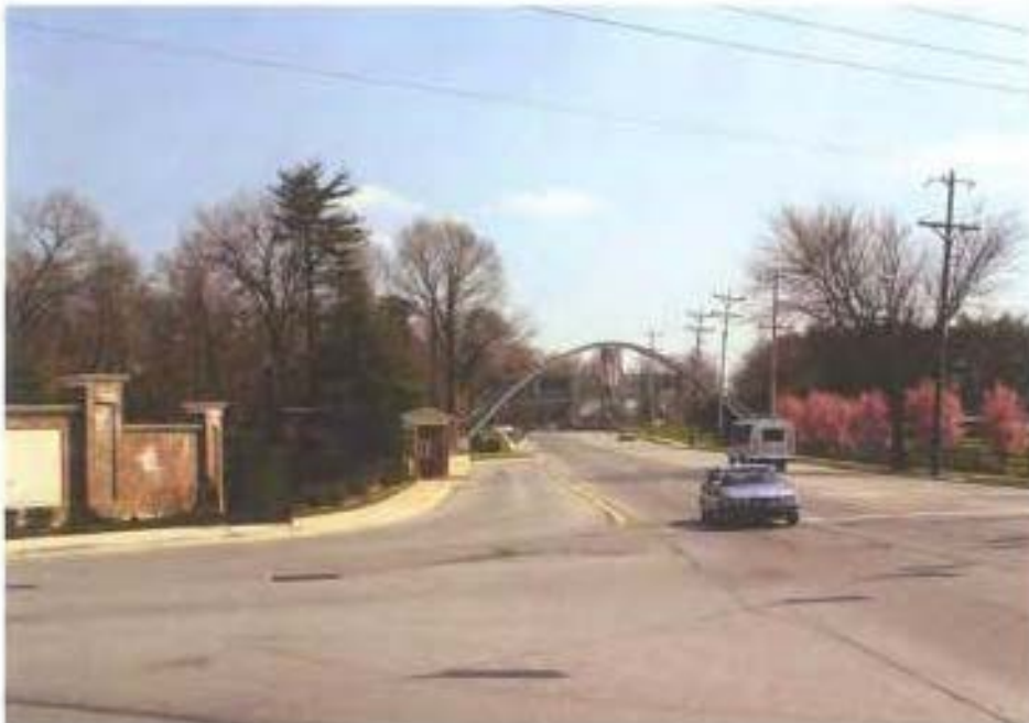
Plate 034 Tower Hill pedestrian overpass on Pennsylvania Avenue
