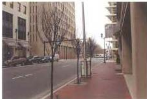
Plate 008 Tree pit conditions on 11th Street
