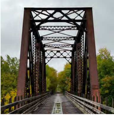
▲ ABOVE: Soo Line Bridge, Palisade
