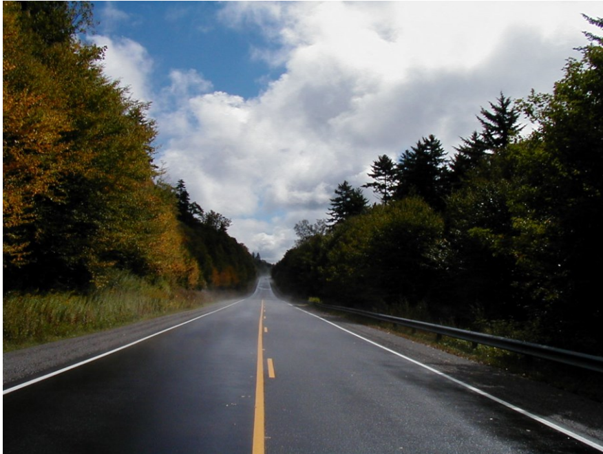
Figure 7 Stretch of Road on HSH/WV 150
