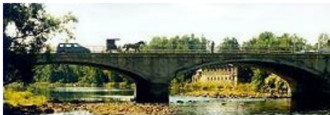
Heuvelton, NY – Present day historic bridge over the Oswegatchie River.
